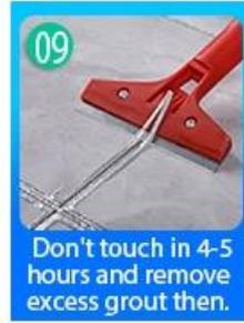
Don't touch in 4-5 hours and remove excess grout then.
